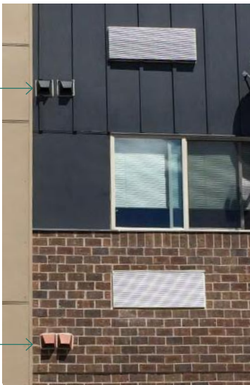
Figure 70.5.Q-16. Utility Appurtenances located on Facades
