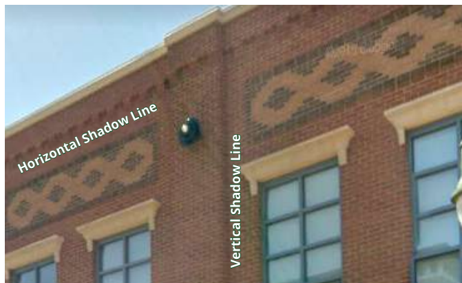
Figure 70.7.A-7. Examples of Shadow Lines
