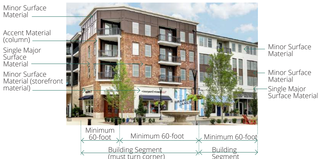
Figure 70.5.Q-1. Major and Minor Materials on a Facade
