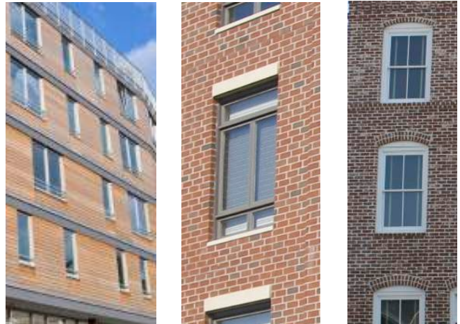
Figure 70.5.Q-7. Vertically Oriented Windows with Expressed Lintels
